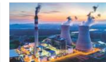
Yadadri - Thermal Power Plant
