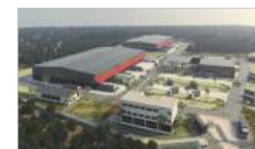
Batasingaram Logistic Park
